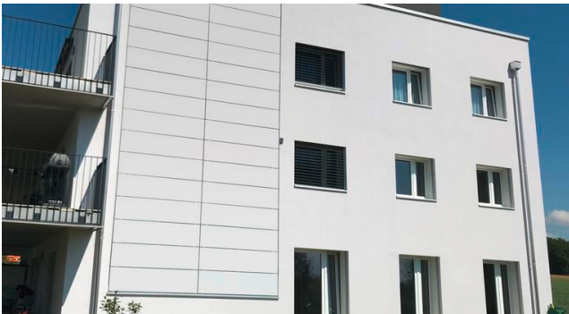
Fig. 2 The photovoltaic panels covering this facade were made by Solaxess (Neuchâtel) using CSEM technology (©Solaxess).
