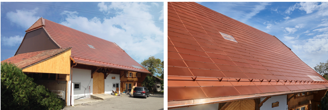
Fig. 1 Renovation project with large terra cotta tiles on a farmhouse located in Ecuivlens (Fribourg, Switzerland) (©Patrick Heinstein).
