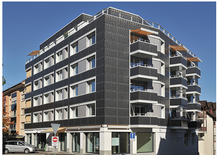
Fig. 2 Renovation of a residential building in Romanshorn (©Viriden + Partner).
