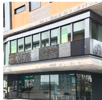
Fig. 4 PV railing at NEST@empa (©HSLU-CC-EASE).
