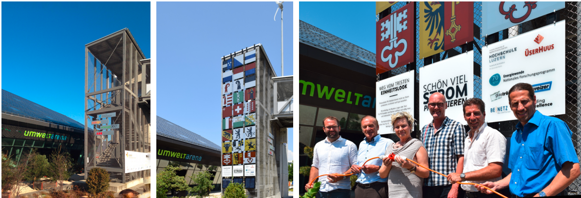
Fig. 2 Original staircase tower (left) retrofitted with Swissness PV facade (middle) and collaborators Walter Schmid (Umweltarena, 2.f.l) and Jacqueline Schindler (ÜserHuus) during its inauguration on 22.06.2017 (©HSLU-CC-EASE).
