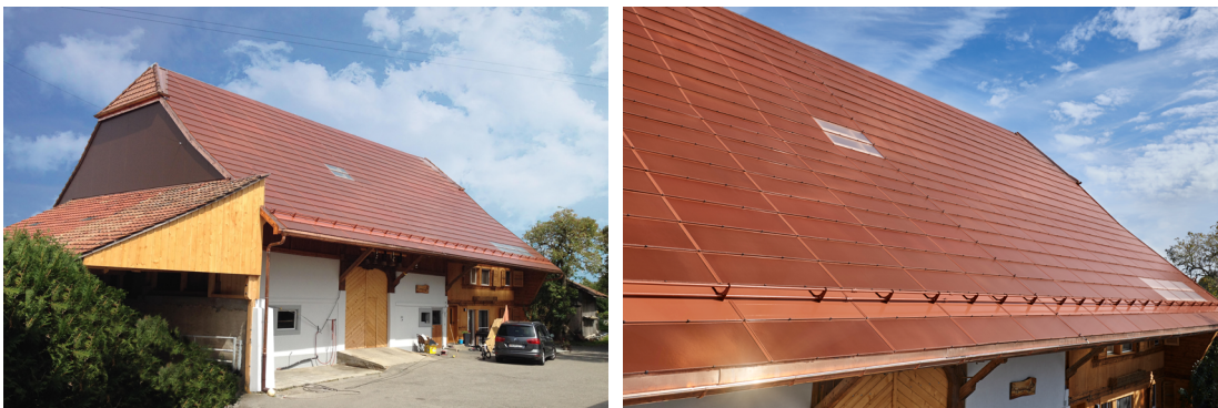
Fig. 1 Renovation project with large terra cotta tiles on a farmhouse located in Ecuivillens (Fribourg, Switzerland) (©Patrick Heinstein).
